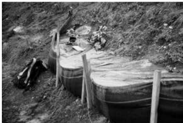
Fig. 6. Eroded sediment accumulated upslope of a silt fence installed following the Bitterroot Fire in 2000 in Bitterroot National Forest, Montana, USA (photo courtesy of Kevin Spigel).
